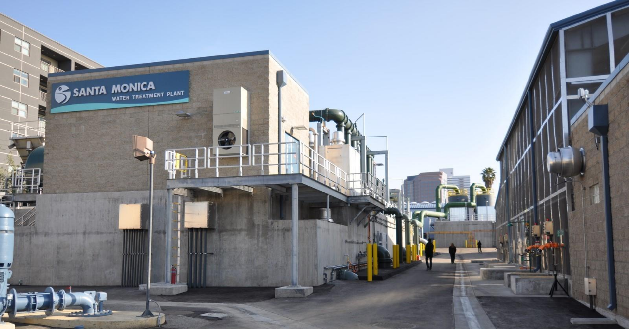
Olympic Well Field Restoration and Arcadia WTP Expansion
