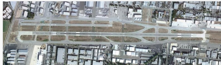
Van Nuys Runway 16R Rehabilitation
