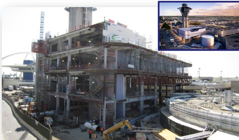
Central Utility Plant (CUP) Replacement Project
