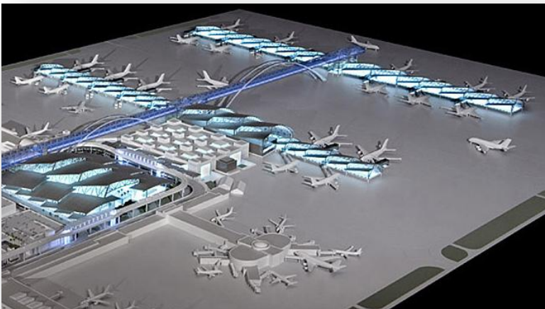
Midfield Satellite Concourse (South)
